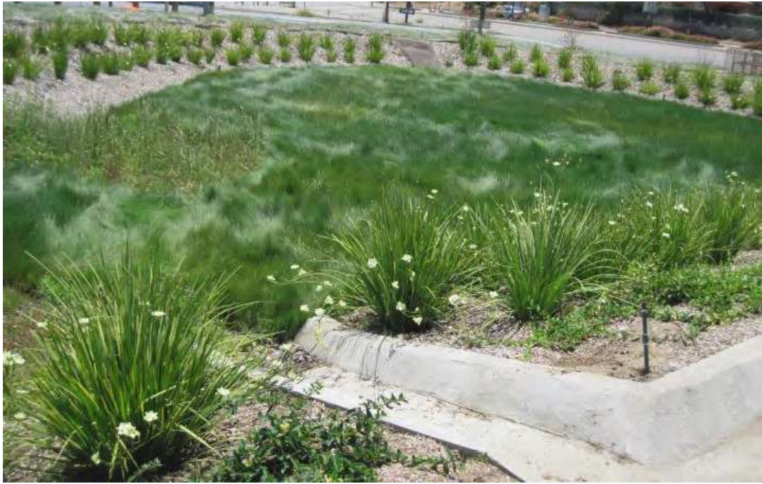
Figure 16: Bio retention area treating highway runoff (Source: Low Impact Development Handbook, Country of San Diego)
